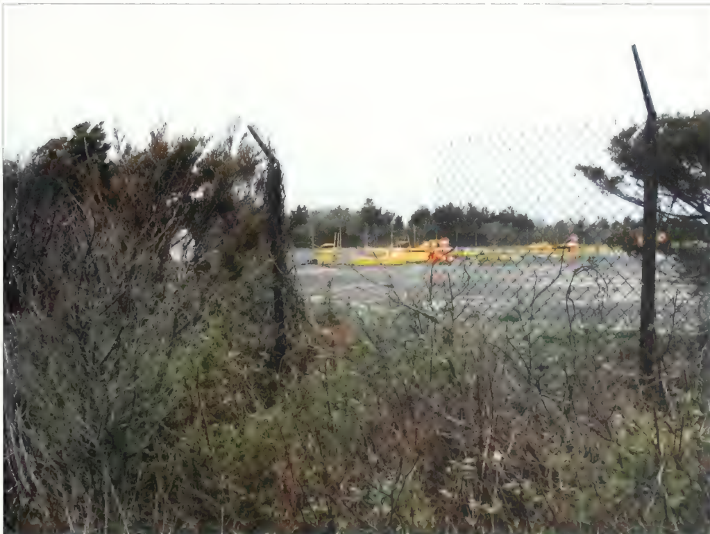
Figure 5.117. View looking east at the missile magazines, NIKE launch site. In contrast to the historic image, extensive vegetation has grown up between the inner fence and perimeter road around the magazines. The dense vegetation will impede repairs to the historic fence (Olmsted Center, April 2008).
